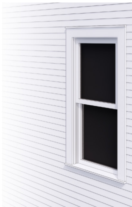
Raised trim should surround windows in walls clad in siding.
