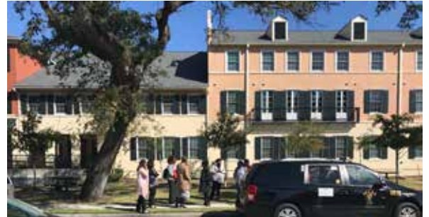
Vertical and horizontal articulation; well-composed windows
