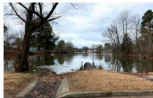
Retention Pond nearly at the same elevation as the road—extremely subject to flooding.
