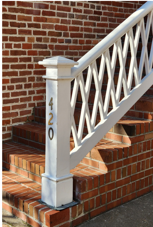
example of existing railing
